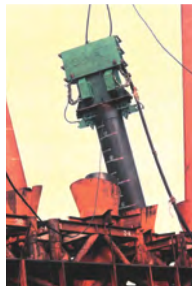
Figure 3: Vibratory hammer.
