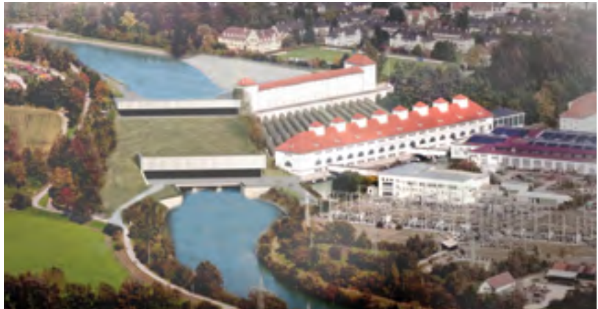
The new Töging power plant is being built right beside the existing historic power plant. Image: Verbund.
