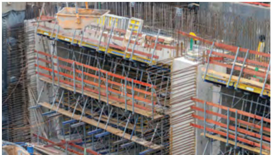
Outlet structure: The outlet structure guides the water back into the Inn river. In addition to the Framed formwork Framax Xlife and Load-bearing tower Staxo 100, Dokamatic tables were used as slab formwork. Image: Doka.
