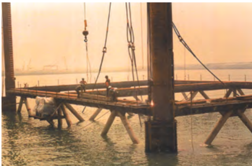
Figure 1: Piling frame.
