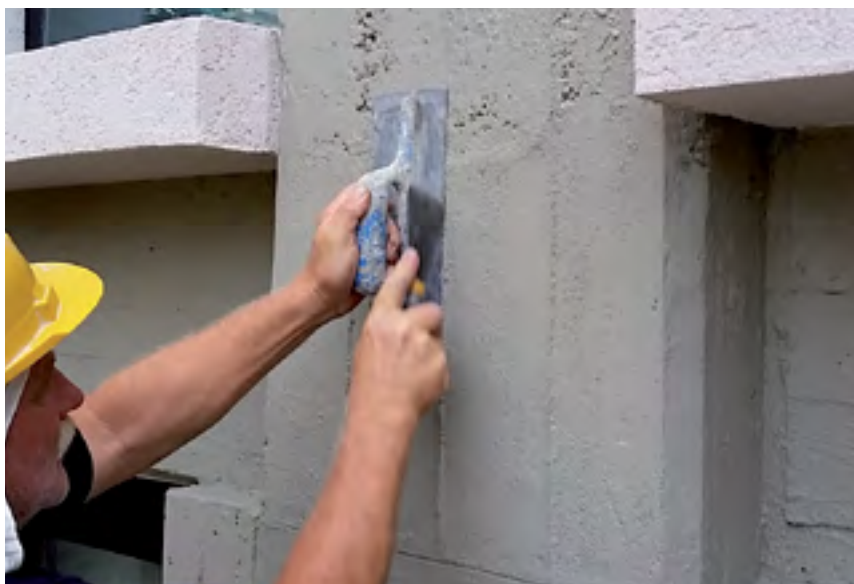
The concrete surfaces of the ledges were skimmed with PLANITOP 210 water-repellent, normal-setting, fine-grained cementitious mortar.
