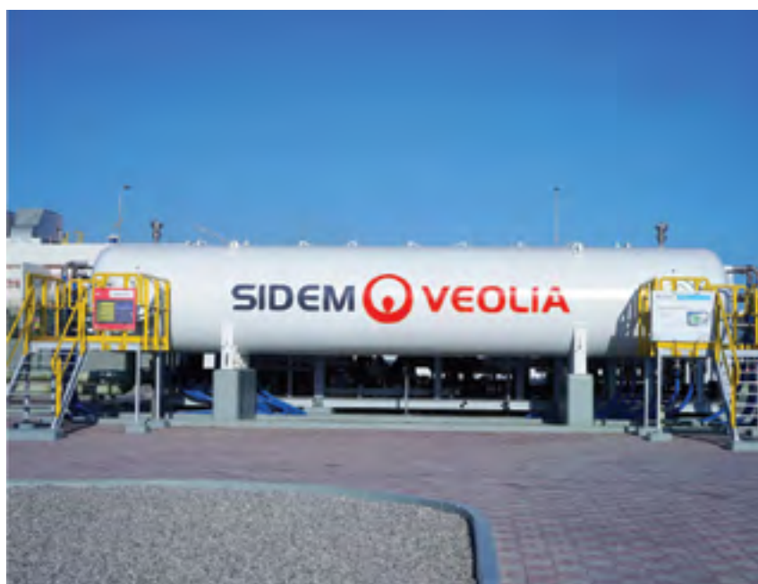
The Barrel is suitable for outdoor installation.
