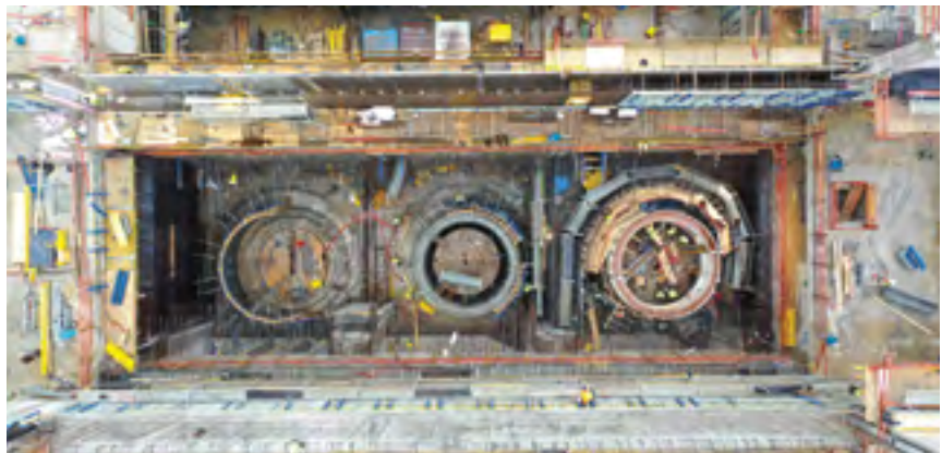
Powerhouse: The main challenges when constructing the powerhouse with its three truncated cones for the turbines, including spiral covers, were the complexity of the cone geometry and turbine slabs, and the ambitious schedule. On top of that, the activities of the numerous participants had to be coordinated. The comprehensive 3D models were extremely helpful for coordination and approval. Image: Kasjan Choroba.
