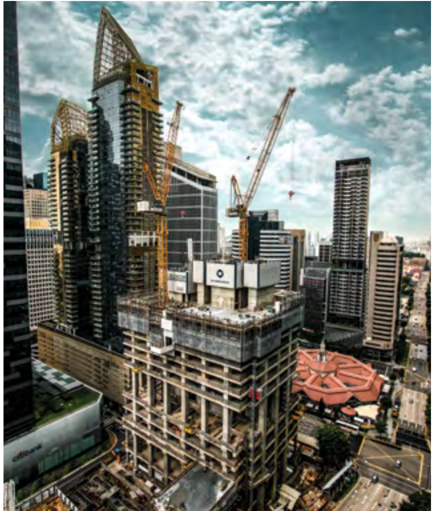
Two Liebherr luffing jib cranes are currently working on the construction of one of the two towers in the Central Boulevard Towers project in Singapore.
