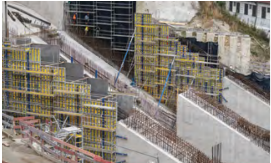
Pressure pipe area: The water plunges down through three pressure pipelines, each with a 10.4 m x 12.75 m cross-section and a gradient of 26.5°. Then the water is directed towards the three Kaplan turbines. Framed formwork Framax Xlife was used to build the steeply inclined walls. Image: Doka.
