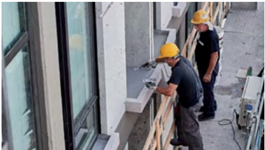
The deteriorated concrete ledges were repaired with MAPEGROUT 430 preblended, normal-setting, fibre-reinforced, thixotropic cementitious mortar.
