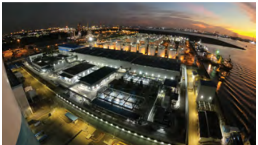
Aerial night-view of the Jurong Island Desalination Plant. Image: PUB, Singapore's National Water Agency.
