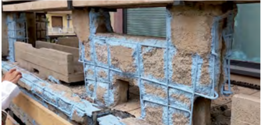
The damaged rebar was protected by applying, by brush, two coats of MAPEFER 1K corrosion-inhibiting cementitious mortar.
