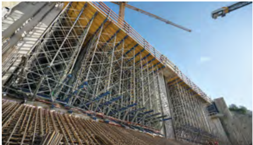
Inlet structure: The water of the Inn river is guided from the inlet structure through the pressure pipeline to the turbine. Around 1,400 frames of the Load-bearing tower Staxo 100 were used for the inlet structure. In order to compensate for the longitudinal incline of 26.5°, the shoring system was installed on a special construction of the Large-area formwork Top 50. The top of the inlet structure was formed with pre-assembled and largely reusable Top 50 elements. Image: Doka.
