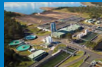
The Prospect Water Filtration Plant in Sydney, Australia.
