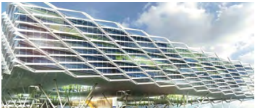
iTWO was used in the cost estimation for the complete shell construction in the World of Sports Arena building project. The steel work consisting of 9,500 tons of steel was completely modelled and estimated in iTWO.
